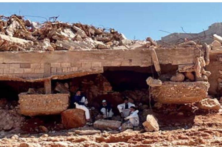
A team of Libyan rescuers rests in the shadow of a collapsed building.
