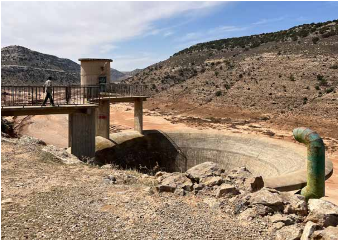
The control tower and the overflow spillway of the Wadi Bu Mansur dam are seen still standing on days after heavy rain caused the collapse of the dam and in turn the catastrophic destruction of Derna, September 2023.
