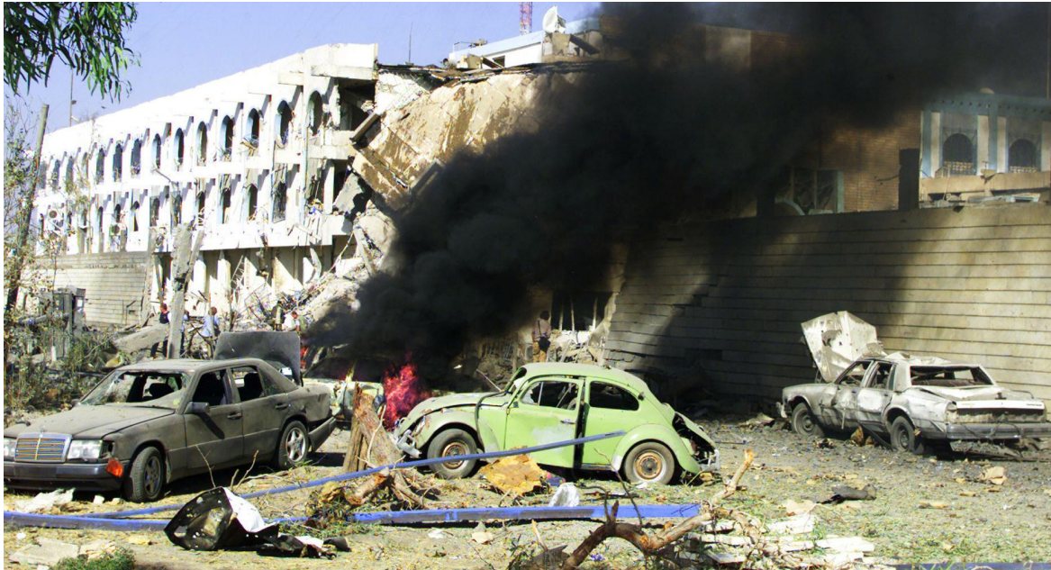
A car burns outside the UN headquarters at the Canal Hotel after a huge suicide truck bomb explosion rocked the building. Baghdad, Iraq, September 2003. AFP PHOTO/Sabah ARAR
