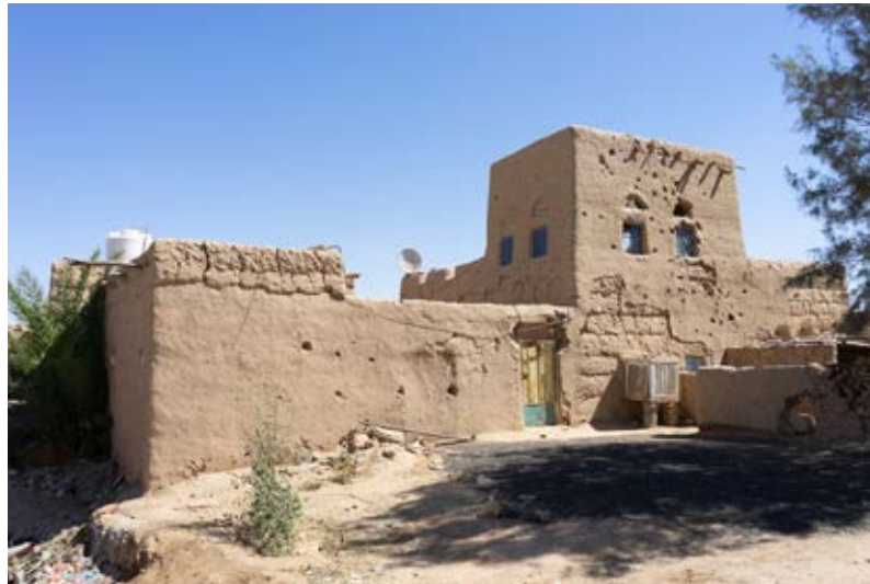
Traditional Yemeni mud-brick house in Serwa.
